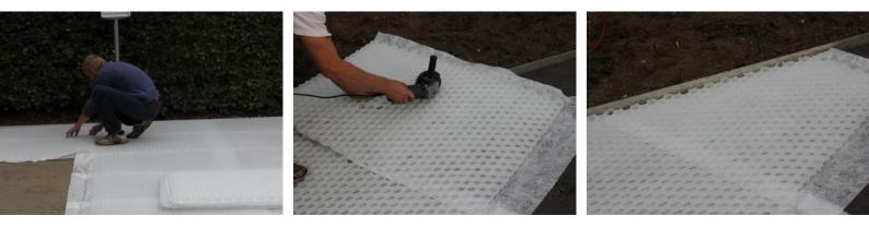
Step 1. The panels are placed on the prepared sub base. Each panel has projecting flaps of membrane. Subsequent panels should be laid on these overlaps to inhibit weed growth between trays and aid product stability.
