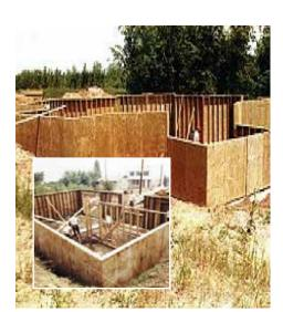
Permanent Wood Foundation (PWF) System is a treated plywood and lumber foundation that installs in any weather. Builders have discovered advantages to include: savings in scheduling; installation by carpentry crews; reduction in material costs, especially where concrete is at a premium, and easy to insulate and finish as a conventional frame wall. The PWF system is all about quality, strength, ease of installation and comfort.
