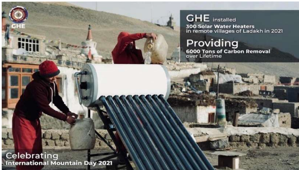
Figure 2: Installation of Solar Water Heaters in Ladakh by GHE Team
