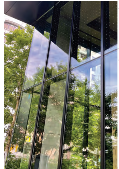
The greenery-facing windows of 1 Hotel Brooklyn Bridge were treated with Feather Friendly bird-safe film. The dots on such window treatments must be spaced closely enough that birds perceive an impenetrable barrier.
