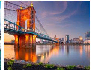
SEP John A. Roebling Suspension Bridge, Cincinnati, OH
