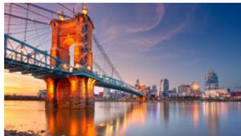
SEP John A. Roebling Suspension Bridge, Cincinnati, OH
