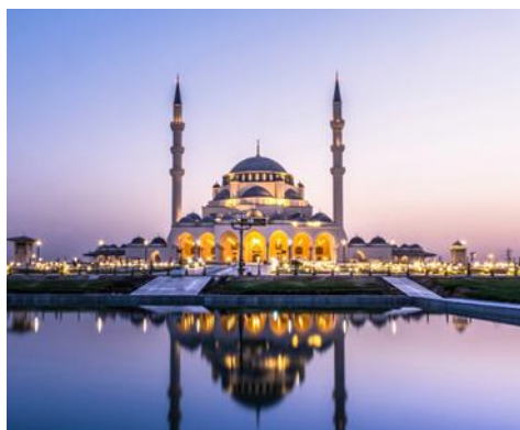
NOV Sharjah Mosque, Emirate of Sharjah, United Arab Emirates
