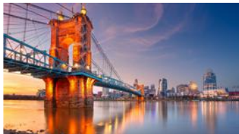
SEP John A. Roebling Suspension Bridge, Cincinnati, OH
