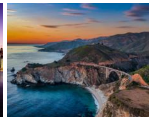
DEC Bixby Creek Bridge, Big Sur, Monterey County
