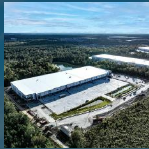
NORTHGATE INDUSTRIAL - BLDG. 3 RINCON, GA 31326
