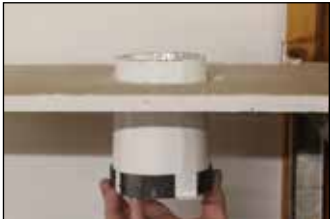
Take unit and push into prepared hole in ceiling/wall.
