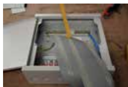
SCU/B Intumescent back gasket which will protect the cable entry from the back and seal off in the event of a fire.
