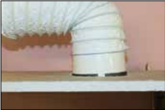
Flexible pipe can be pulled through the hole, rested onto the CLVM & pushed up into the ceiling
