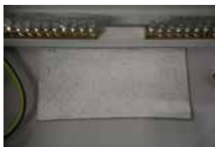
SCU/B Intumescent back gasket which will protect the cable entry from the back and seal off in the event of a fire.
