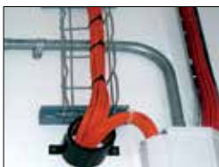
WPCS COLLAR CAN BE USED FOR CABLES
