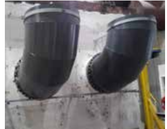
EXTERNAL VIEW BEFORE TEST
