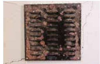
MGL Grille inside the furnace after the fire test
