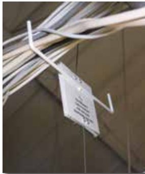
Cables laying on top of the suspended ceiling - serious evacuation hazard
