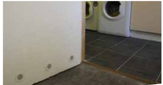
Laundry Room Installation
