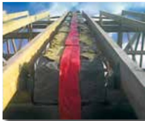
Cavity seal fixed in cavity roof section: Projected verge using gable ladder
