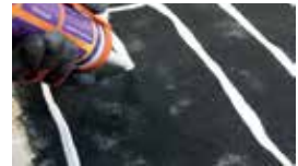
Generously spread the adhesive on the surface of the sponge.
