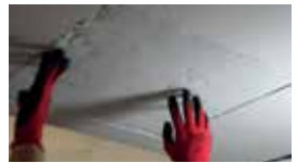
Assure a good contact and leave for 2 hours. You can then staple the material to the lathes if required
