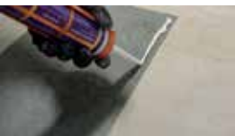
Generously spread the adhesive round the overlapping edges .
