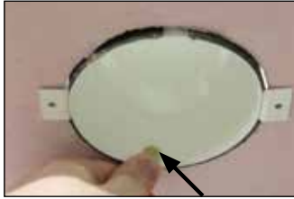
Fasten in position with supplied pins, 2 to side and 2 in the bottom holes.
