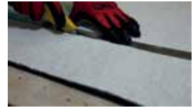
Cut the sponge to size and shape of the created hole.
