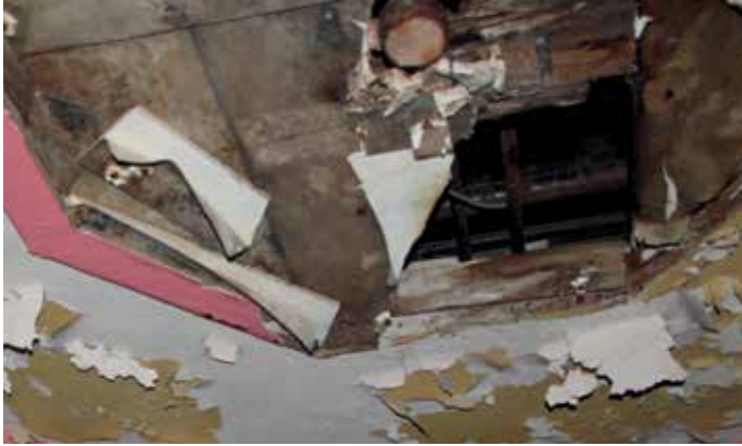
Clean off any loose parts of the plaster and measure the hole.
