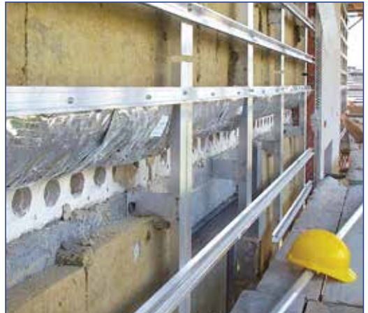
Flexible mesh structure
