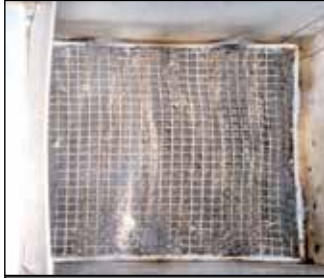
BLOCK GRILLE IN DUCTING AFTER A FIRE TEST
