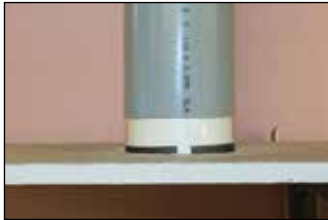
Slide the PVC or flexible PVC pipe down the unit.
