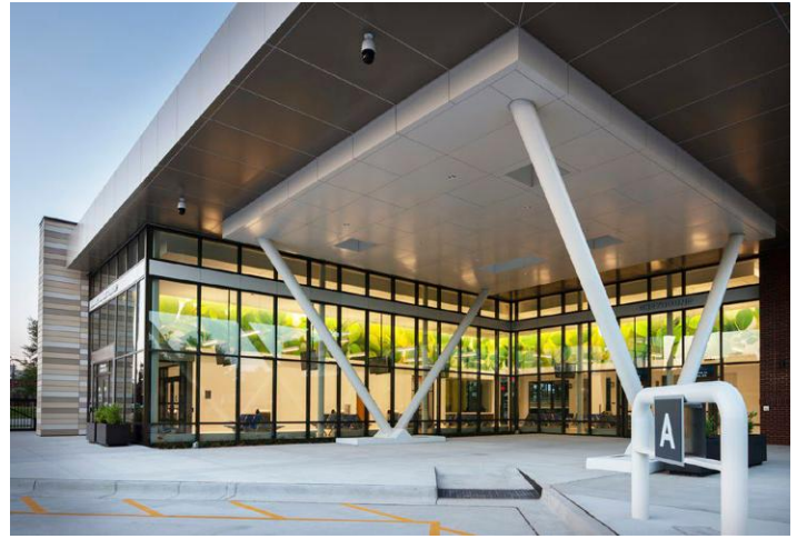
ALBANY TRANSPORTATION CENTER ALBANY, GEORGIA
