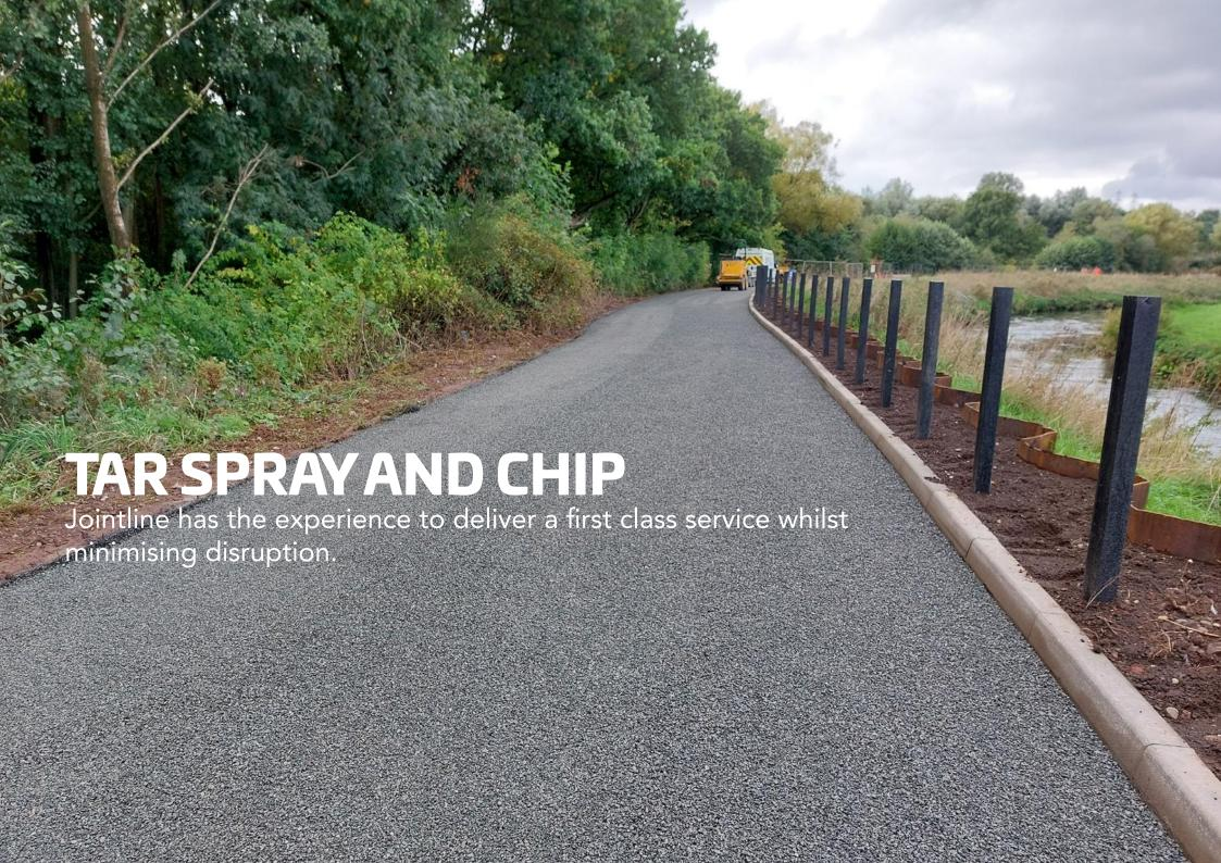
A durable surface dressing binder, tar and chip surfacing is a low-cost alternative to asphalt and is ideal for producing a high quality, natural and aesthetically pleasing finish to drives and footpaths for commercial and large residential projects. Jointline install either a hot applied or a cold applied surface dressing binder that is suitable to the clients requirements and dressed with a range of decorative coloured aggregates.
