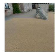
Resin Bonded Surfacing System provides an attractive, hard wearing and low maintenance surface by bonding or fixing loose gravel aggregates to concrete, asphalt, wood or metal.
