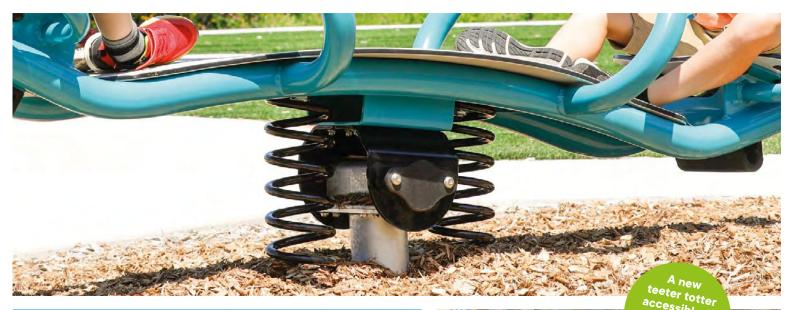
Two coil springs developed specifically for Jambette by a major Canadian manufacturer provide the rocking motion of the Silla–2 rocker. They are pinch-free for hands and feet. The top end of each spring is fastened to the underside of the equipment platform, while the bottom end is secured to the underground anchoring system by simple design mounting brackets that stand the test of time.
