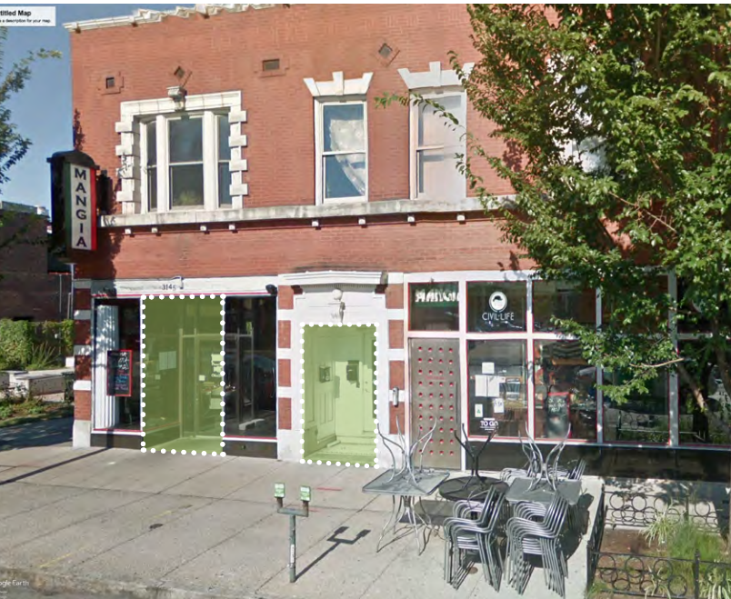
Ground-floor entrances are recessed to avoid door swings in the pedestrian walkway, photo by Google.
