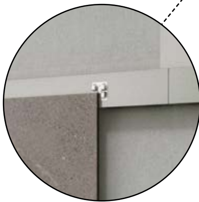
Dettaglio gancio AM Detail of harmonic steel hook
