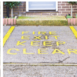
Fire Exits: "No Parking"
