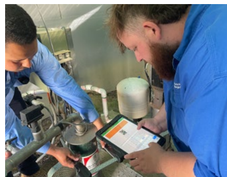
NRAR outreach officers inspecting a pump during an on site visit. Photo: NRAR
