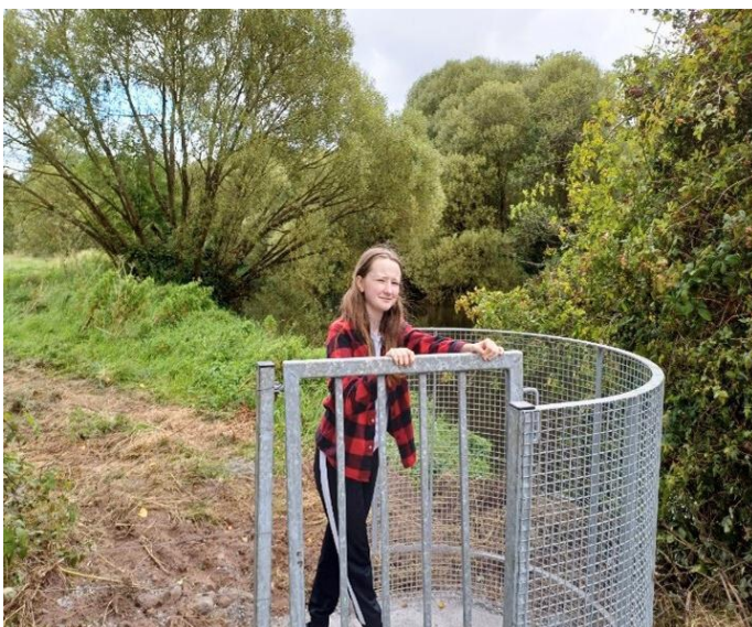
A new kissing gate installed at Suirville
