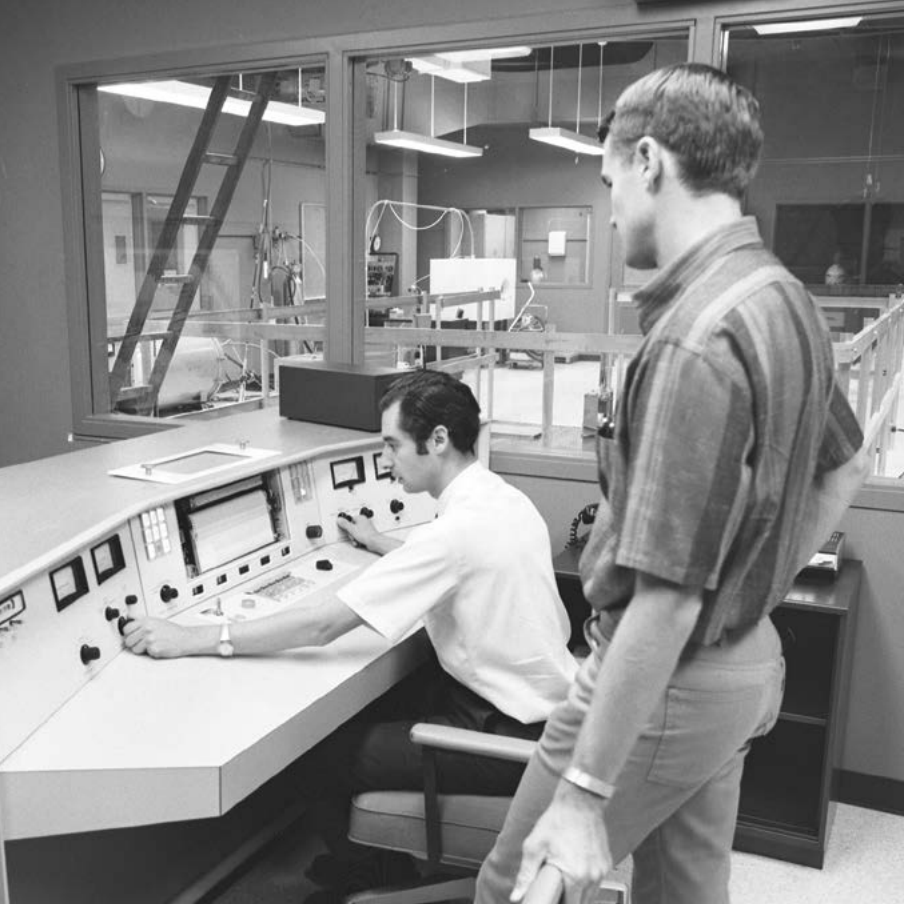
Professor George Miller and Pat Grant check the reactor's console, UC Irvine Nuclear Reactor Facility, 1969
