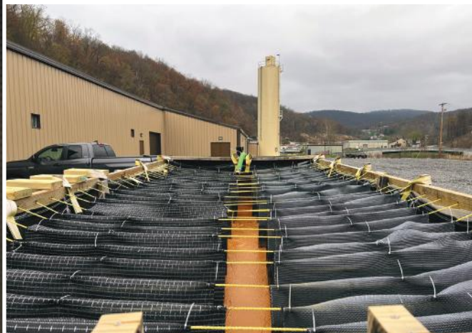
This mobile system at an acid mine drainage site in Morgantown, West Virginia, extracts water from soil on site rather than transporting it to a lab.
