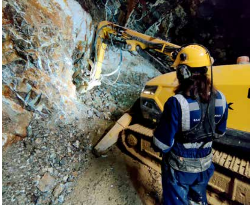
The versatility of remote-controlled demolition machines can minimize equipment and personnel requirements for highly efficient renovation.
