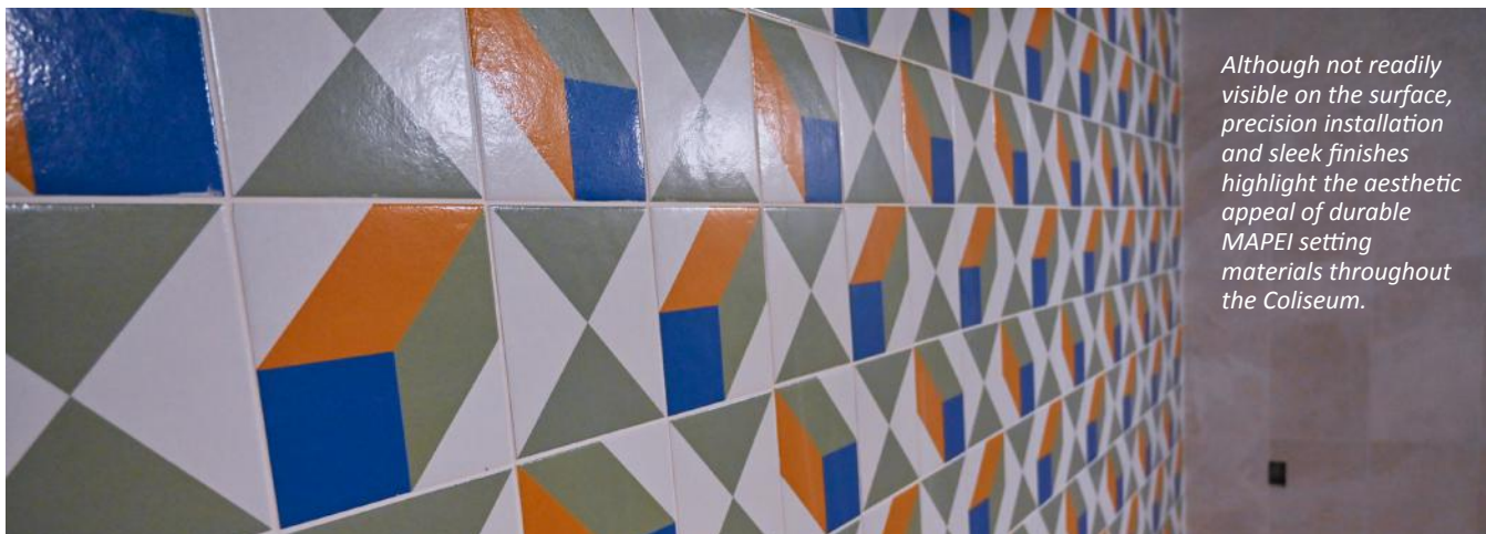
Tile awaiting grouting with MAPEI's epoxy grout Kerapoxy CQ. This grout was chosen for application throughout the building for its stain resistance, durability, and easy maintenance.
