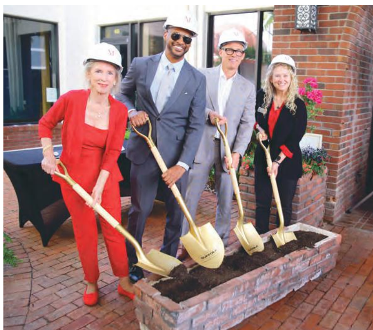
Celebrating the groundbreaking of Mira Mar Residences on South Palm Avenue on May 20 are, from left, Brenda Patten of Berlin Patten Ebling; City Commissioner Kyle Battie; Patrick DiPinto, principal of Mira Mar Acquisition Company; and City Commissioner Jen Ahearn-Koch.
