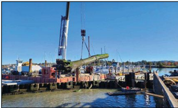
The contractor removed the large tree from below the fishing pier as part of the in-water work.
