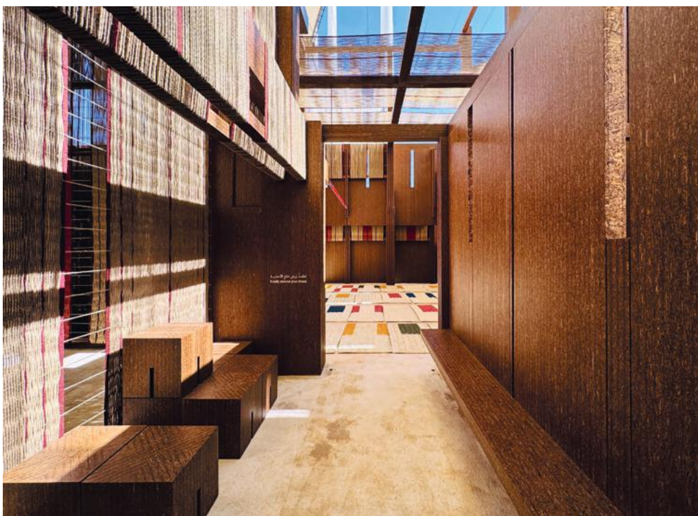
Below The modular structure allows reuse and is intended to resemble a loom; gaps in the facades filter and diffuse daylight.
