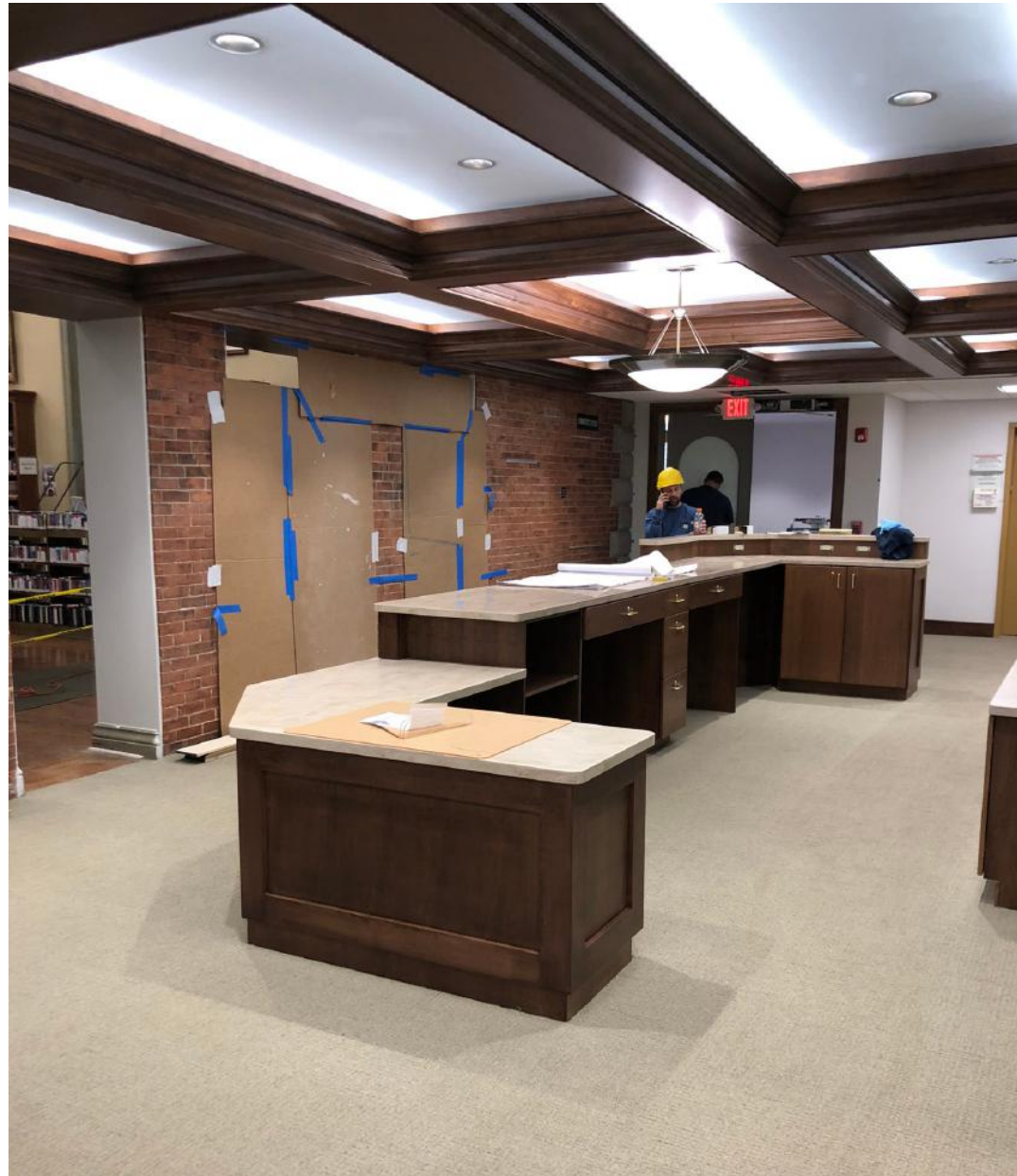
FIRST FLOOR CIRCULATION AT CONSTRUCTION
