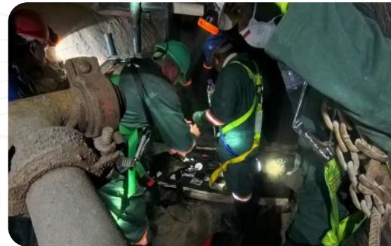
Image: The GammaTec crew preparing the Elios 3 before launch – showing how confined space inspections can now be done safely without risking personnel underground
