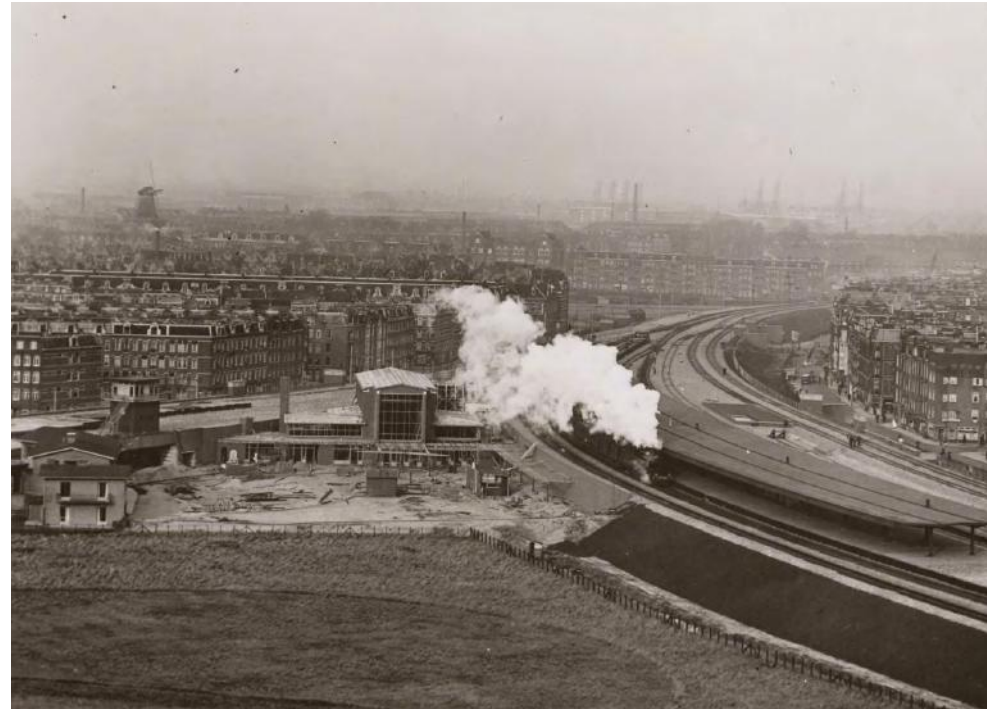
Station Muiderpoort in aanbouw, 1939. [SAA]
