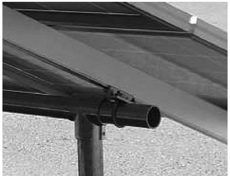
Attach Pipe Mount to Rail
