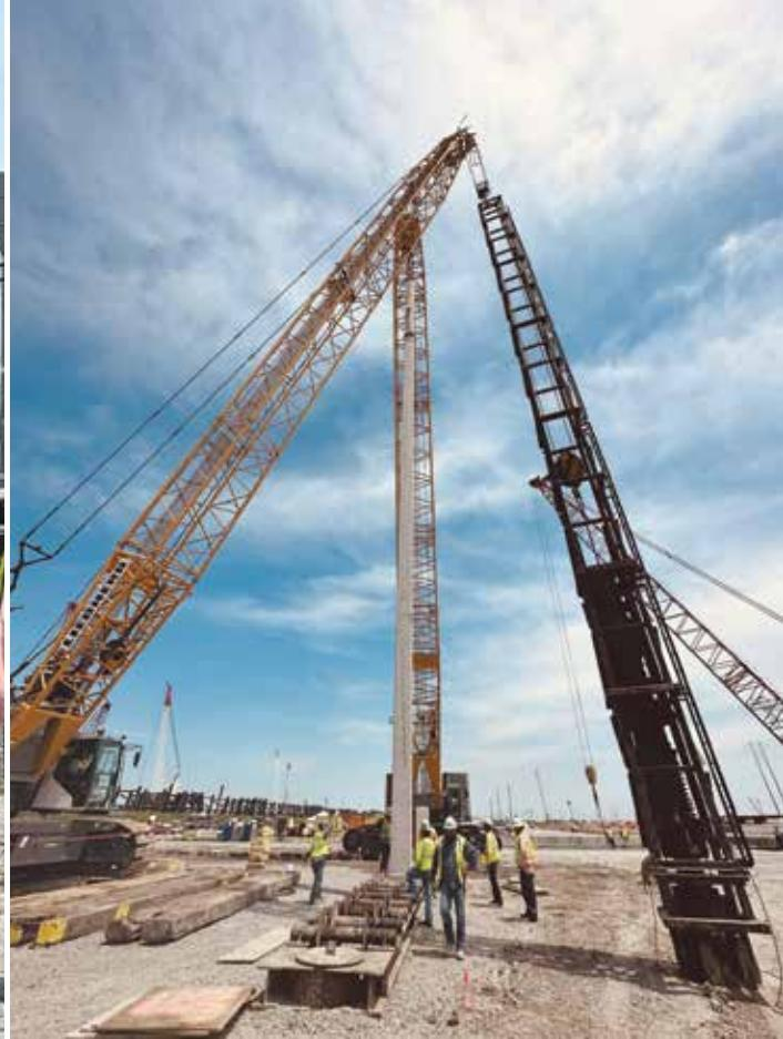
Each set of eight piles required six compression tests, two tension tests and two lateral tests.
