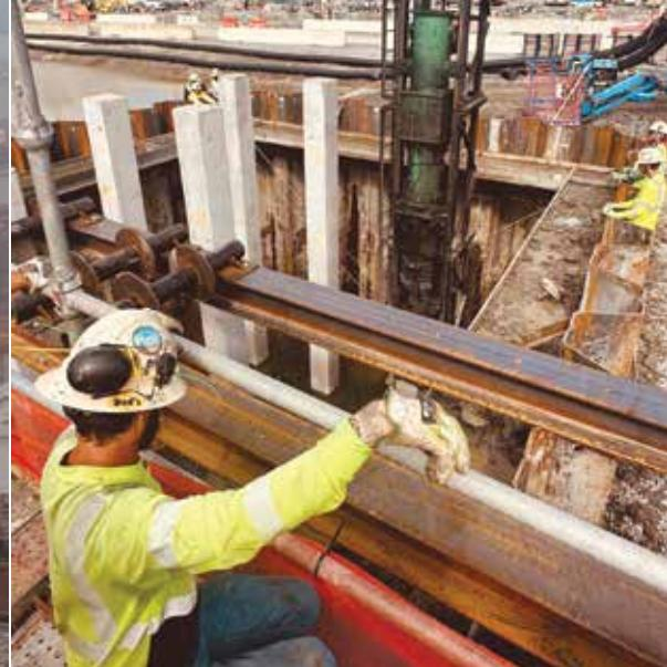
faced numerous logistical hurdles including managing the delivery and placement of massive steel sheet piles and coordinating the installation of floodgates and other structures while other construction activities were starting to ramp up. The successful execution of this scope was a testament to the team's expertise and commitment to project success.
