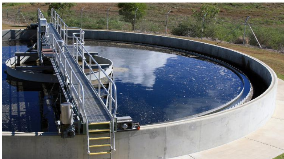
Farm irrigation water pump (top) and water treatment plant (above) Images: Supplied Pampsix & Gomez David
