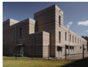
Boiler House, St. Petersburg. Architects: Lenenergo, St. Petersburg Seite / Page 246
