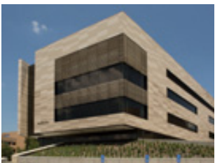
University of Kansas, Earth, Energy & Environment Center. Architects: Gould Evans, Lawrence, KS Seite / Page 56
