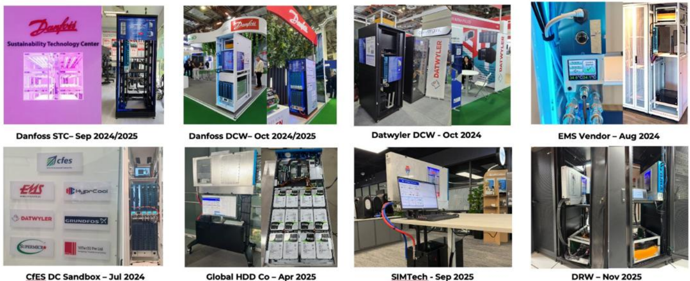
Figure 7 – Standalone SJI Liquid Cooling System installed at various customer premises
