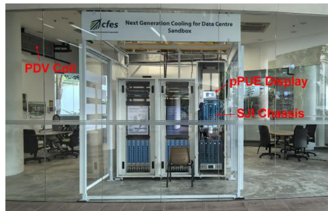
Figure 4 – SJI Liquid Cooling cum PDV Pilot Systems at Ngee Ann Polytechnic
