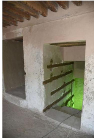
Schematic sketch of needling in the staircase pier
