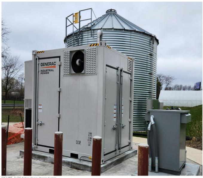
FIGURE 3-04 Battery Energy Storage System.
