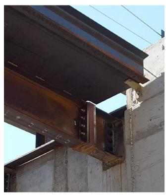
FIGURE 3-16 Thermally broken steel detail.
