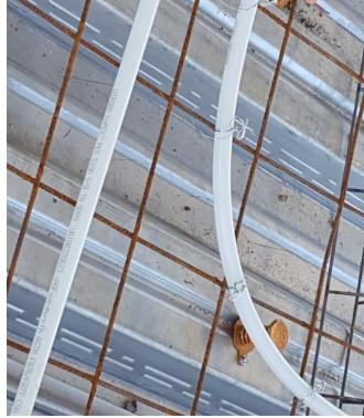
FIGURE 3-17 Detail of Radiant Tubing.
