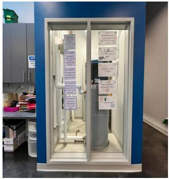
FIGURE 3-02 Heat Pump Hot Water Heater.
