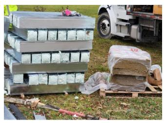
FIGURE 5-04 Insulated CFMF headers on site.
