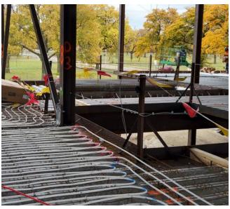
FIGURE 3-12 Radiant Tubing before Concrete Floor
