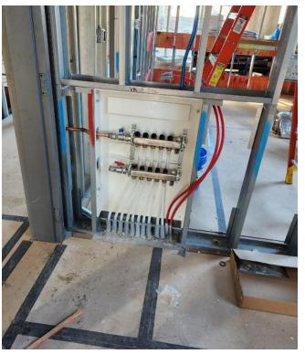
FIGURE 3-14 Radiant Tubing Manifold
