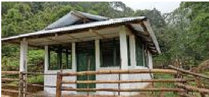
A Community Activity Center (CAC) building in a village in Arunachal Pradesh
