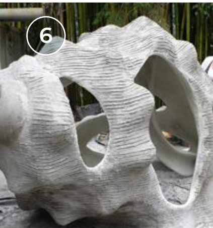
6 GFRC concrete added to frame
