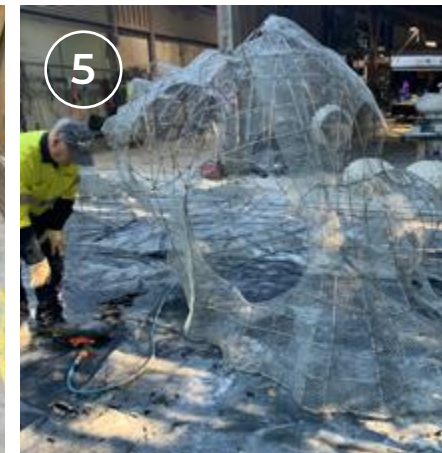
5 Wire mesh over substructure
