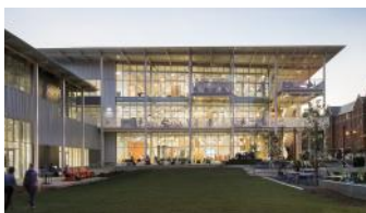
Chapter 7 Construction Details: West Village Dining Commons (WVDC)
