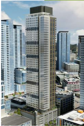
1001 John - Seattle, WA [400 foot, 430 unit residential tower]
