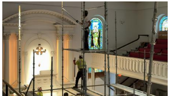
Early work on the interior scaffolding.
