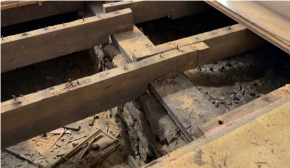
Shoring for the truss repair begins at the ground level - literally!
