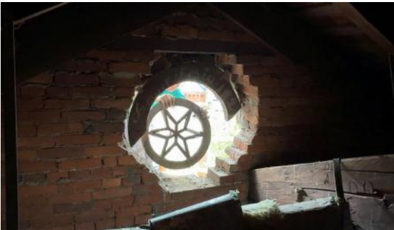
One of the circle windows along Washington Street being removed.
