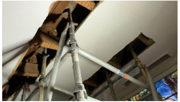
This is what the shoring looks like bracing the balcony above.
