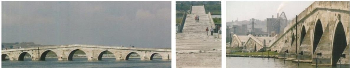
Figure.4. Views from Büyükçekmece bridge, (Necipoğlu G,2005)
