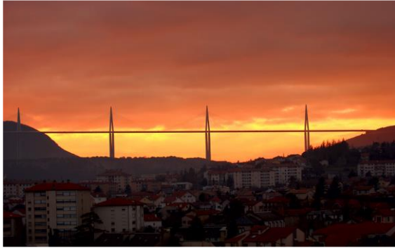
Figure.8. Millau Viaduct, France, 1993-2004 ) ( www.fosterandpartners.com )
