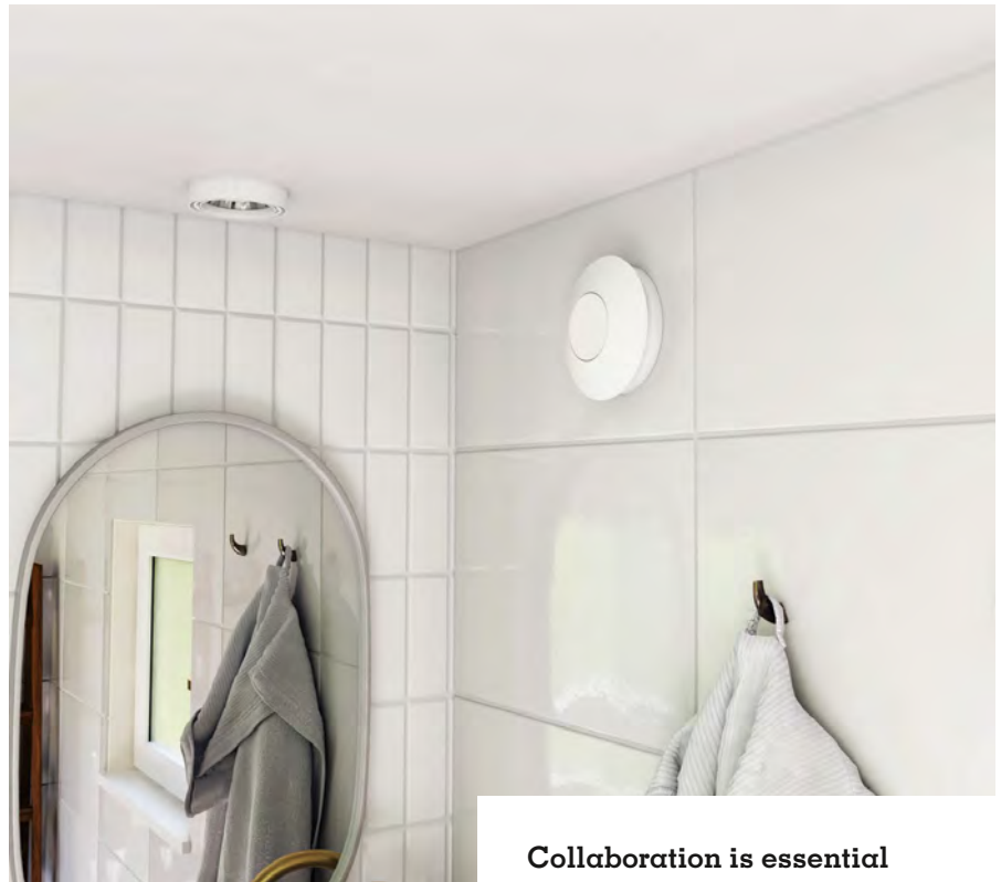
Modern fans can run constantly with an integrated humidity sensor to give a boost or on-demand ventilation when required
