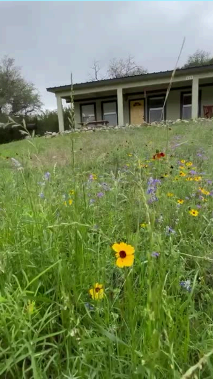
VIEW TO FRONT PORCH
