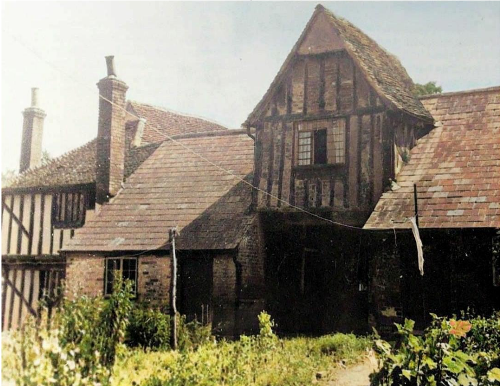
North side before restoration - 1952
