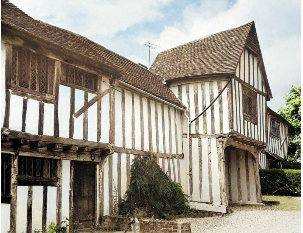
North side after restoration.
