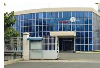
First Factory Building
