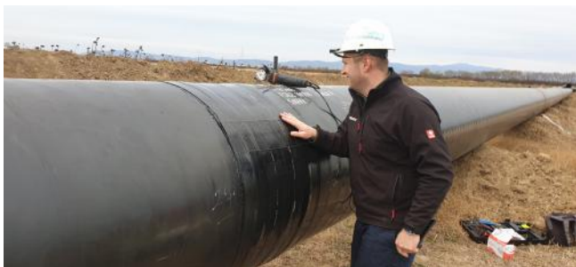
Figure 1. Martin Durcik undertakes an on-site inspection of the coated joint.
