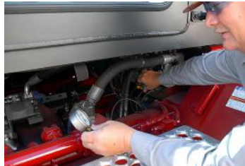
Service & Inspection from Ground Level
