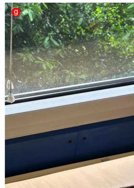
Panelling in living room is easily removable for future inspection
