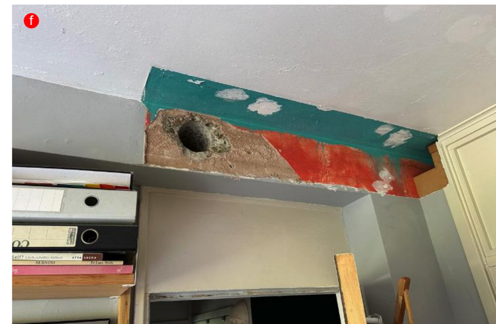
Remnant of historic service distribution, stripped out during renovation
