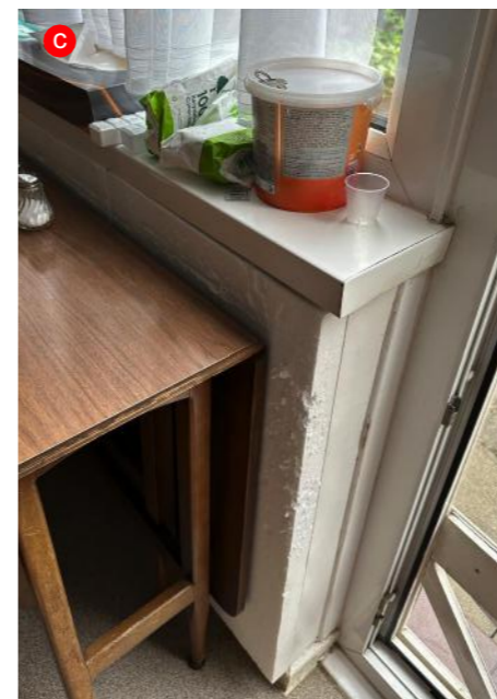
DIY internal insulation to address thermal discomfort in winter
