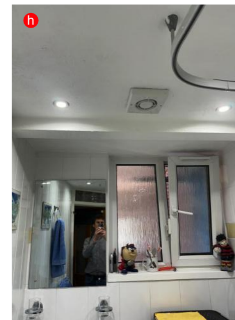
Window to third external elevation and extract fan to exterior in bathroom
