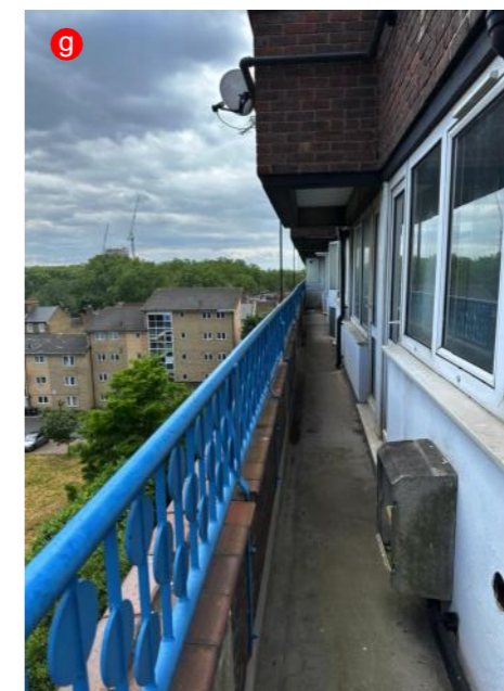
6th floor escape balcony running over living room
