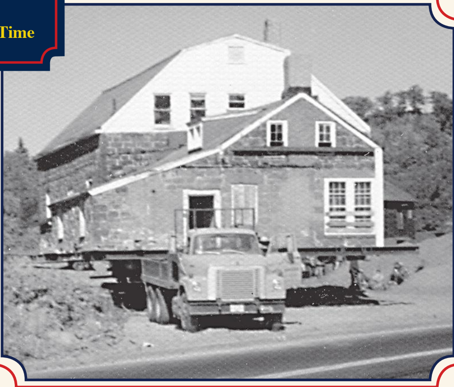
March 4, 1980: The Van Wagoner-Hamilton House was relocated by truck from the Notch on Valley Rd. and moved a few hundred feet up the street to its present location at Surgent Park. These days, the Hamilton House at 971 Valley Rd. is Clifton's living history museum and will be open for tours in June.
