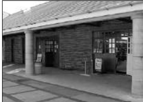
The new Pharmacy and PC shop are located in the courtyard opposite to The Student Centre
