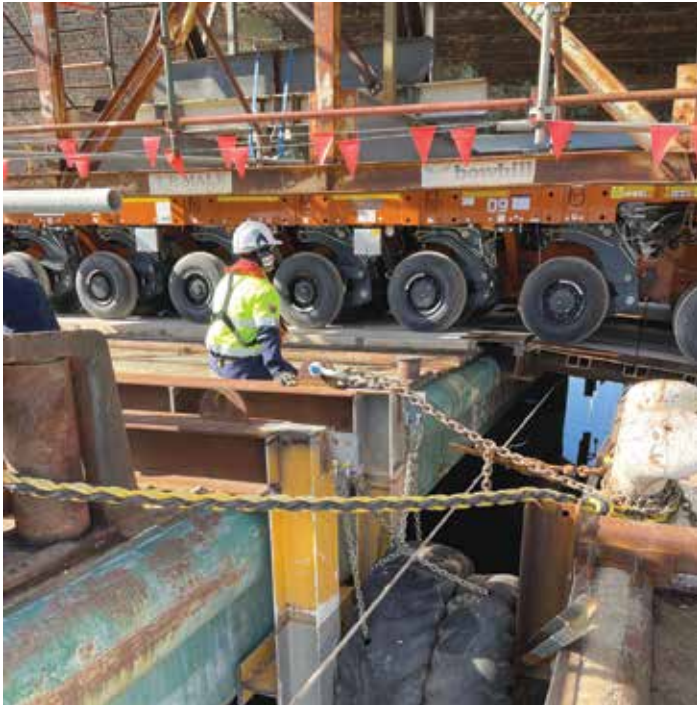
SPMTs carrying cradle and ship from barge to land
