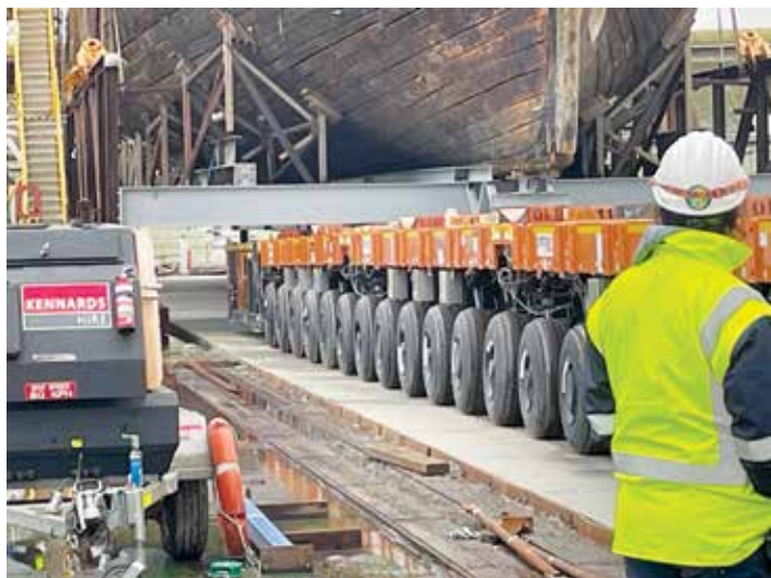
SPMTs driving onto barge under cradle
