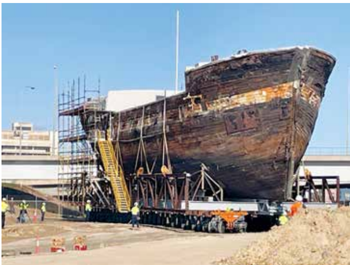
The SPMTs turning to enter Pit
