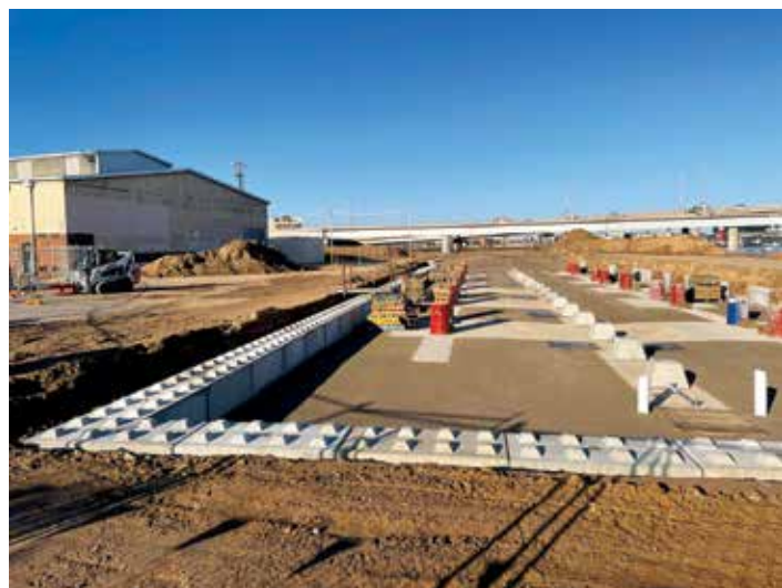
Pit and foundations ready to receive cradle and ship on SPMTs
