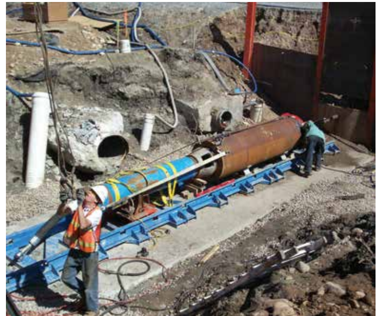
Figure 7.4.1 - Pilot tube guided pipe ram.
