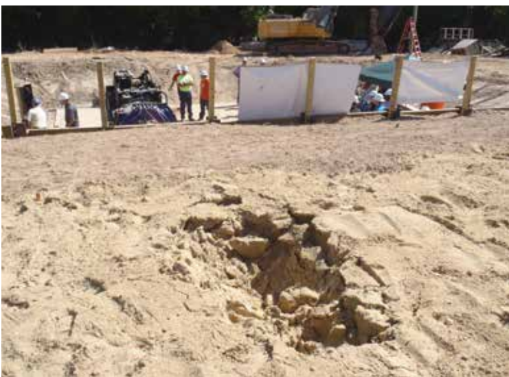
Figure 4.10 Surface settlement in sand section. (Courtesy of TTC Auger Boring School)
