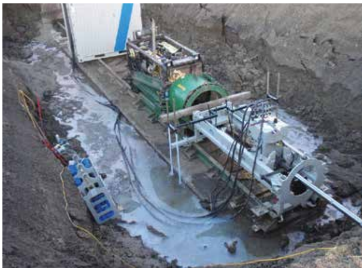
Figure 7.2.3 - Excavated bore pit operation.
