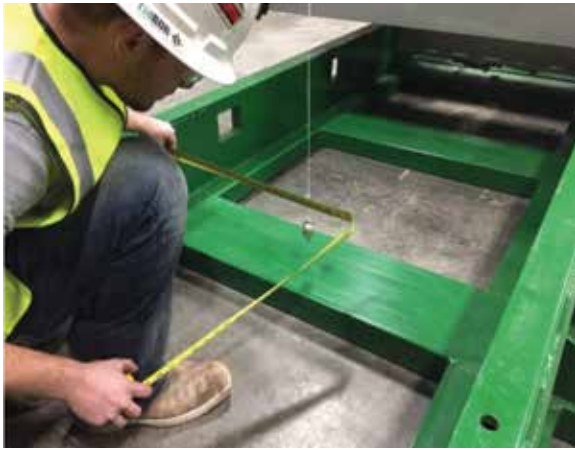
Figure 7.3.1.2 - Machinery centerline is matched to the plum bob.
