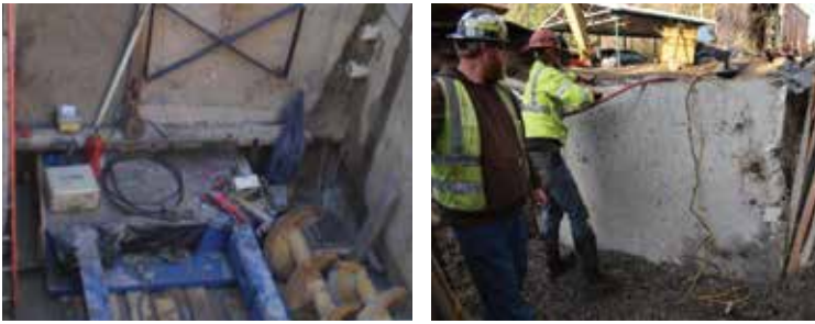
Figure 4.4 Cast in place concrete thrust blocks. (Courtesy of Midwest Mole, Inc.)
