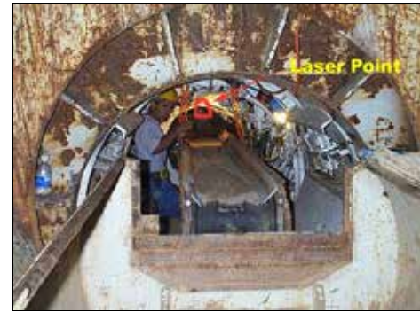
Figure 5.5 Laser guidance system for pipe jacking. (Abraham and Gokhale, 2002)
