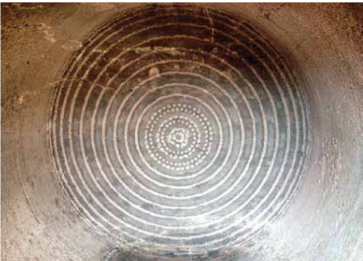
Figure 4.14 Kerf Cutting Pattern in Rock Face. (Courtesy of The Robbins Company)
