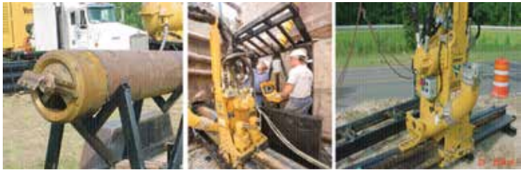
Figure 7.5.1 – VMT components along with jacking set up.
