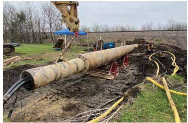
Figure 10.1 Hydraulic leveling jacks being used to support casing for line and grade.
