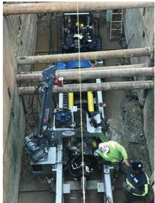
Figure 7.3.1.7 - Stringlines are left in place during operation.
