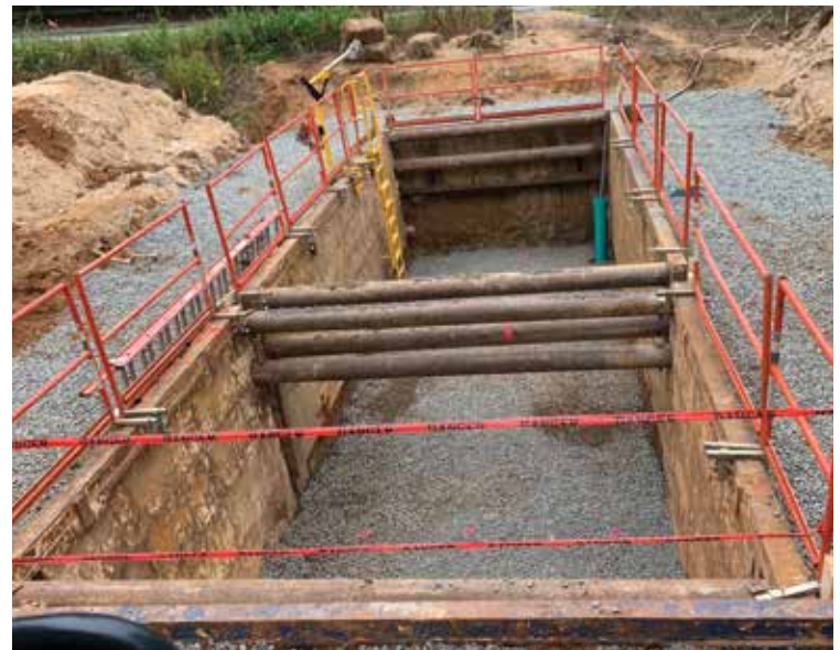
Figure 4.2 The boring pit bottom filled with crushed stone. (Courtesy of Brent Scarbrough Company)
