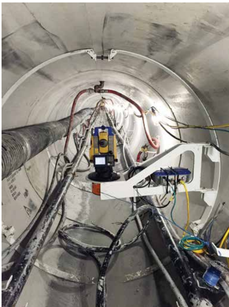
Figure 6.7 Azimuth-Laser Total Guidance System – Tunnel Station.
