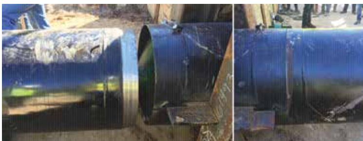
Figure 4.11 The weldless interlock pipe joints system. (Courtesy of TTC Auger Boring School)
