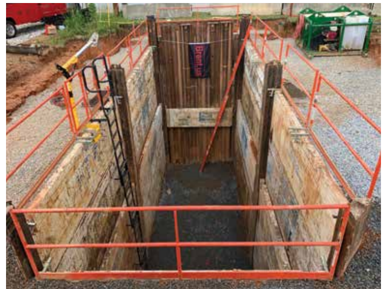
Figure 4.3 The boring pit. (Courtesy of Brent Scarbrough Company)
